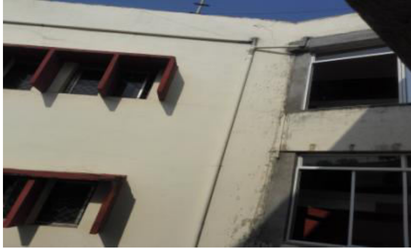
Photograph of Pipe line network for Roof Rain water Harvesting
